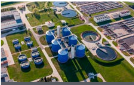
Sewage treatment plants
